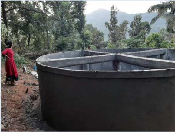
Tank Under construction
